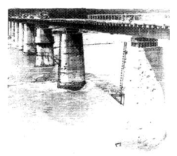
Figure 103. Typical solid concrete pier.
