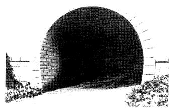
Figure 120. Typical masonry lined tunnel.
