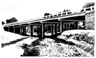
Figure 61. Typical concrete slab bridge.
