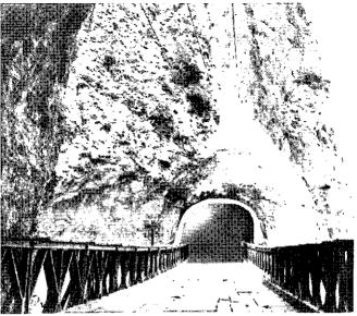
Figure 121. Typical concrete lined tunnel.
