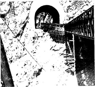
Figure 123. Typical concrete tunnel portal.
