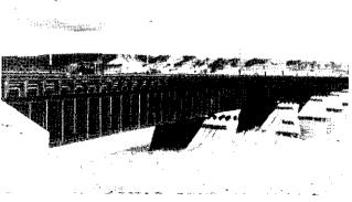
Figure 78. Typical multispan plate girder bridge.
