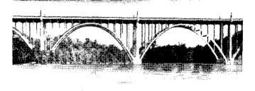
Figure 87. Steel trussed deck arch bridge.
