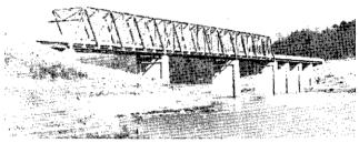
Figure 75. Typical steel through truss bridge (Warren type).
