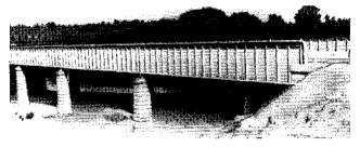
Figure 79. Through type girder bridge.
