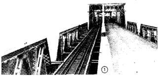
1 Pony truss and through truss forming combination bridge Figure 76. Typical pony truss spans.
