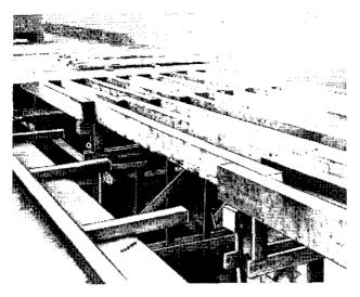
Figure 63. Simple stringer bridge with rectangular timber stringers.
