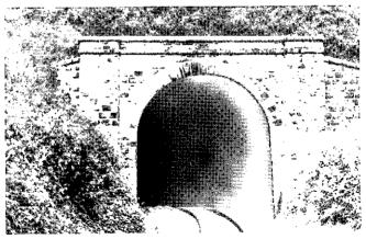
Figure 122. Typical masonry tunnel portal.
