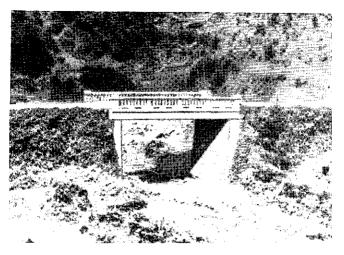
Figure 67. Typical single span concrete bridge.
