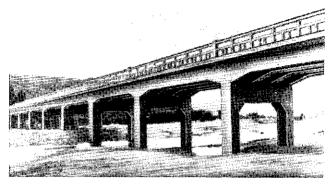
Figure 69. Typical multispan concrete T-beam bridge.
