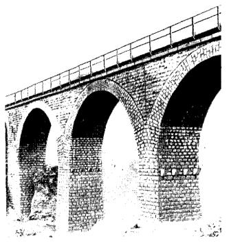
Figure 83. Typical solid masonry arch bridge.
