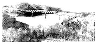
Figure 73. Typical steel deck truss bridge.
