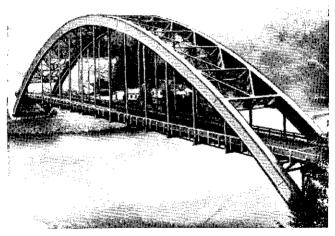
Figure 88. Steel arch bridge, through type.
