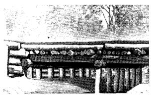
Figure 64. Simple stringer bridge with log stringer.
