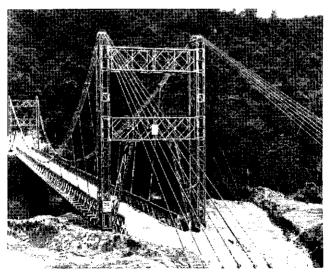
Figure 91. Bailey type suspension bridge.
